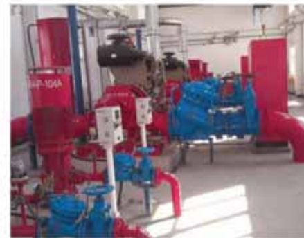
宁夏炼油柴油机消防泵 Ningxia oil refining diesel powered fire pump
