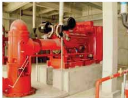
首都机场柴油机立式长轴消防泵组 diesel engine vertical turbine fire pump set in Capital Airport
