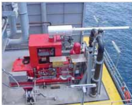
洛克石油柴油机立式消防泵组 Locke petroleum set diesel engine vertical turbine fire pump
